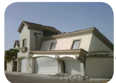
2010: A home in Calexico, CA after the Easter Sunday 7.2 earthquake
